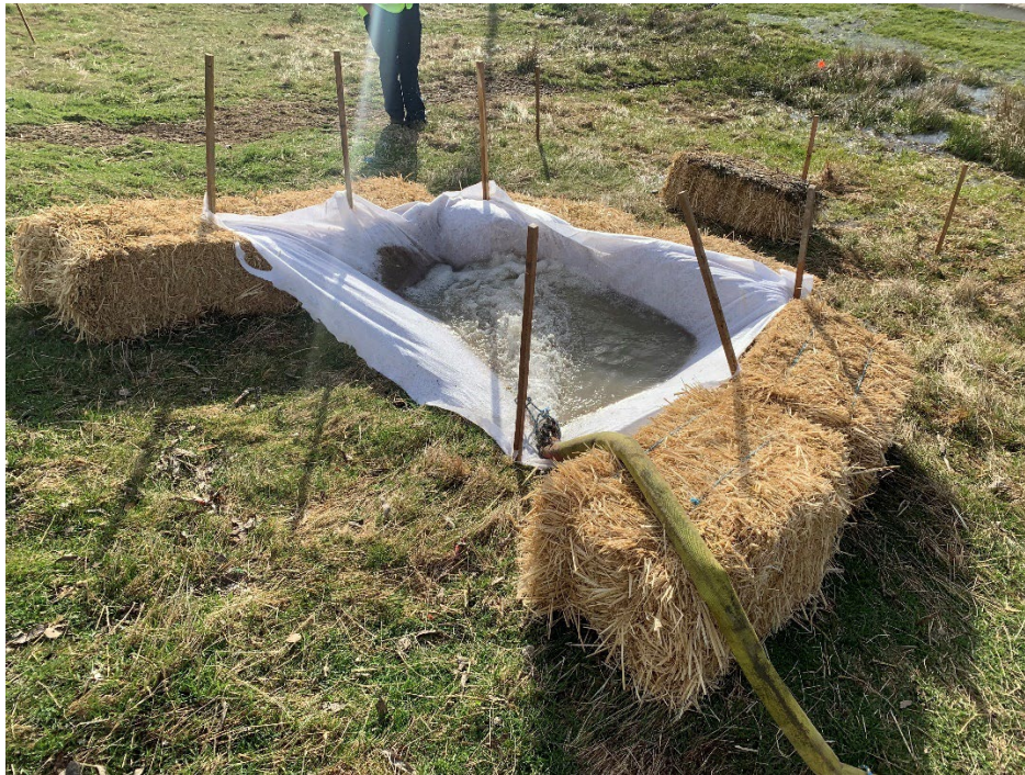
Figure 4: Filter Dam Example
